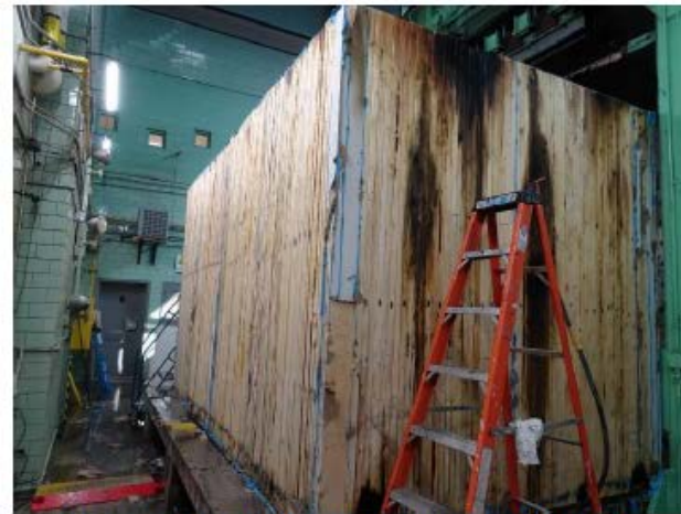
(a) NLT exterior (gypsum board removed)
