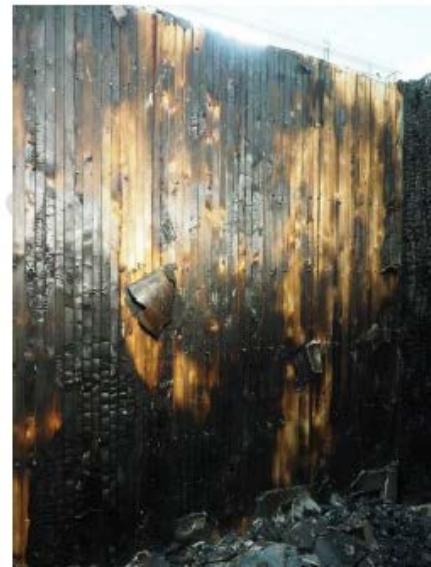
(c) Wall A (interior gypsum board removed)
